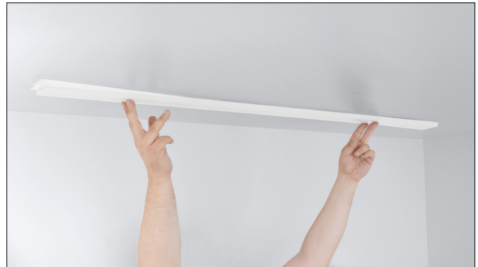
Step 6: Insert lens into light engine to close the luminaire.
