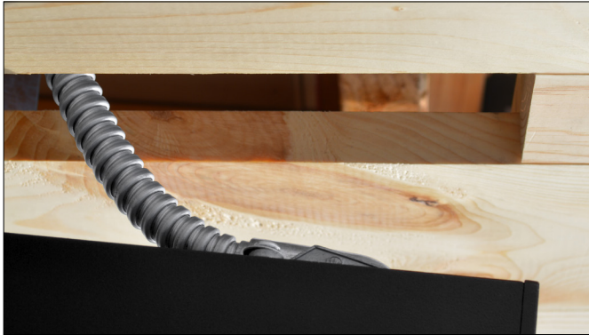
Step 3: Insert luminaire into opening.
