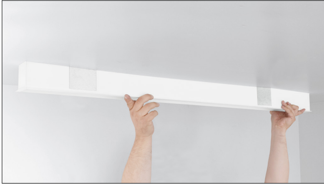
Step 3: Remove lens and light engine from luminaire then install luminaire body in ceiling.
