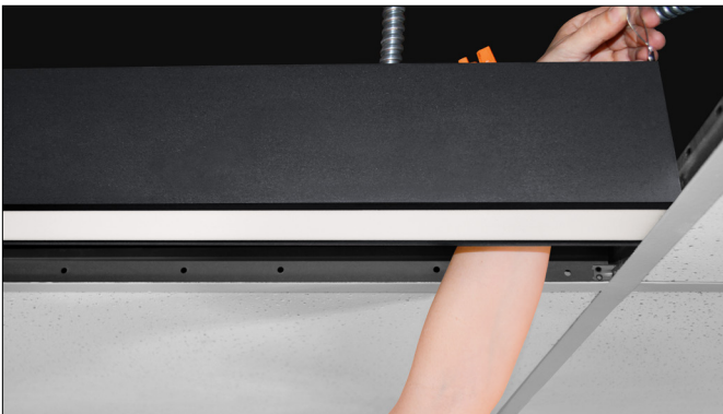
Step 3: Lay Vector luminaire in grid at desired position. Secure Vector to structure above using structural wire (by others) via holes in the Vector 2 end plates.
