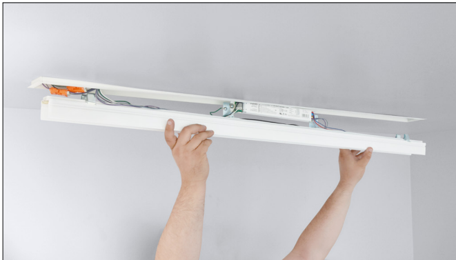
Step 5: Connect light engine using quick disconnects for power and dimming. Snap light engine into luminaire body.
