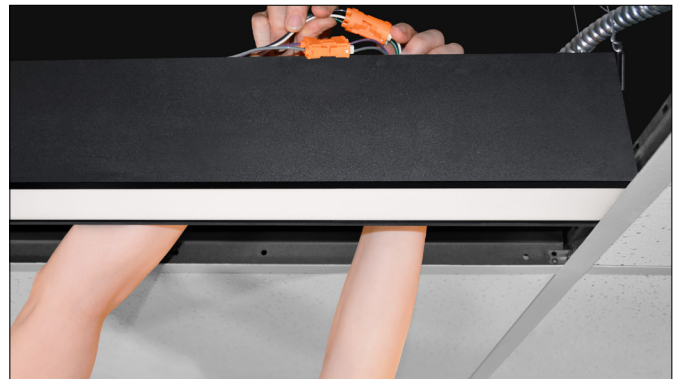
Step 4: Connect pigtail disconnects to luminaire disconnects. Insert wires into housing. Insert knockout plate and fasten using screw provided.
