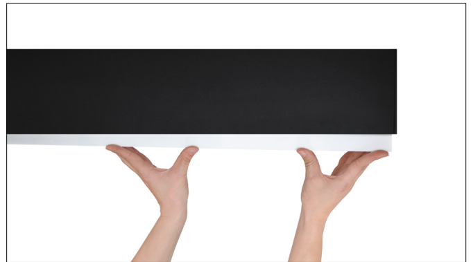
Step 6: Snap tray in place; Snap lens in place.
