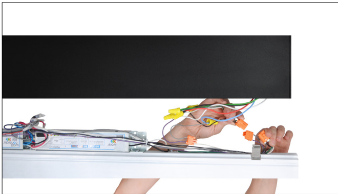
Step 5: Connect tray to power.
